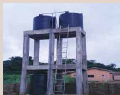
The people of Echara- unuhu, Izzi in Ebonyi state where our postulate House is located lacks portable water. St. Helen's sewing center constructed overhead tank with capacity of 12,000 liters of water and drilled motorized borehole in order for the community have access to portable water.
